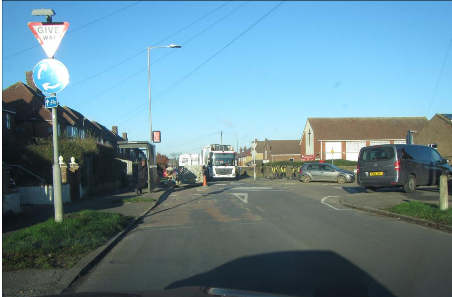
Figure 3 Rutland Avenue just to the north of The Middleway which will become a raised table in the proposals
